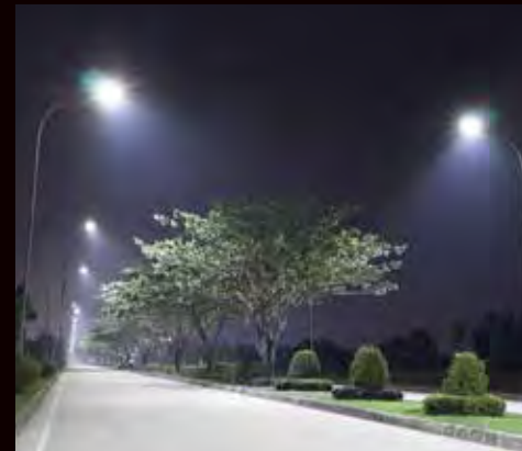
Karawang International Industrial City (KIIC), Indonesia
