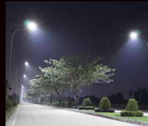
Karawang International Industrial City (KIIC), Indonesia
