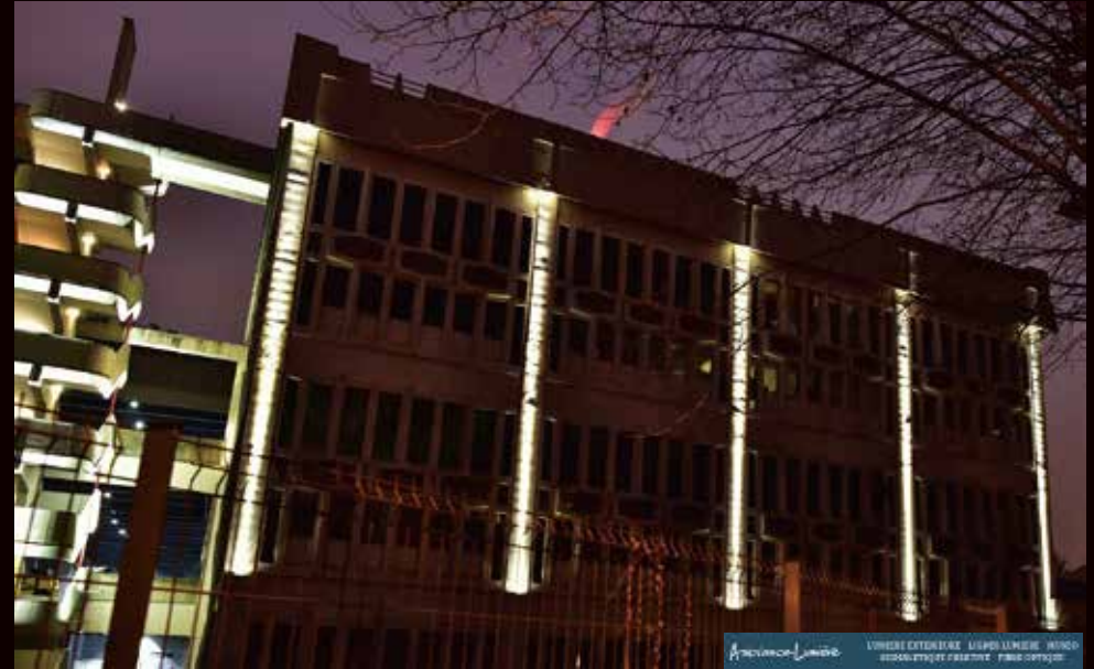
Building in Zone Industrielle de Mozinor in the suburbs of Paris, France
